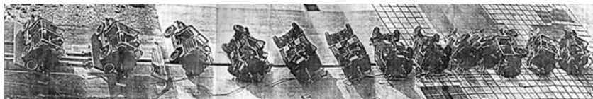
Figure 24. View of the experimental test for the truck rollover.
